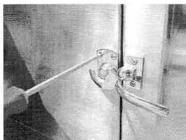
3. By the same way to screw on the screws of the spring bolt (A).
