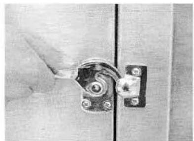
4. Please lock and unlock the door to make sure the lock is not removable and spring bolt (A) and lock catch (B) can be linked with each other.
